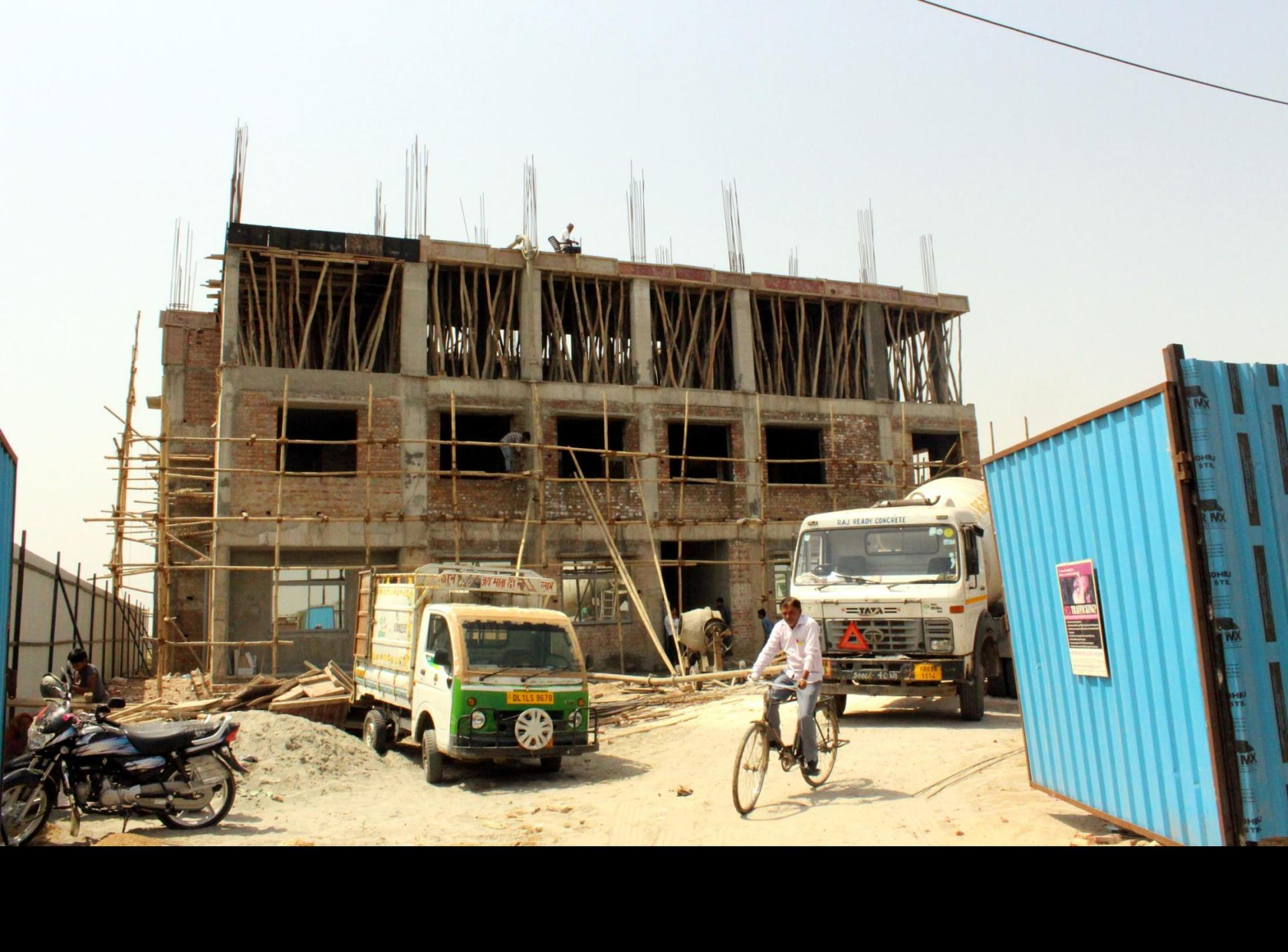
Construction site showing a multi-story building under construction. The structure is partially completed with concrete and brickwork. Scaffolding is visible around the lower levels. The top of the building shows rebar protruding from the concrete slabs. A worker is visible on the roof level.
